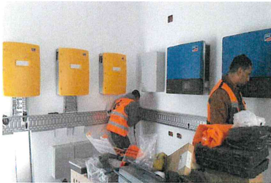
Installation of Inverters
