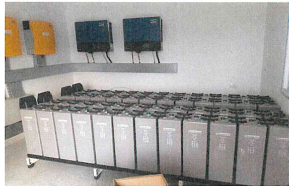
Installation of Batteries
